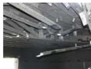
Steel to wood panel point connection failure
