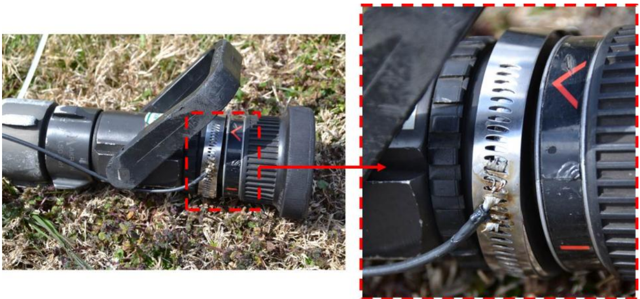
Figure 41 14 AWG stranded copper wire soldered to a hose clamp and affixed to the nozzle's exterior housing
